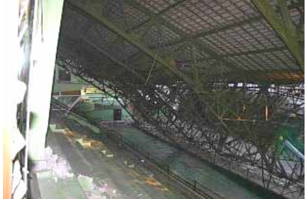
Amongrogo Sport Center / Collapsed roof system associated with column failure underneath
