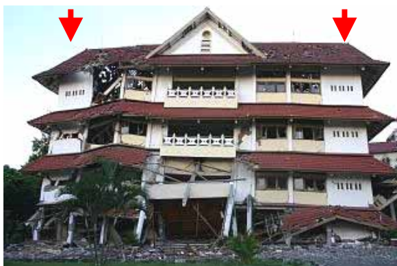
4 story building with 2 URM walls frames
