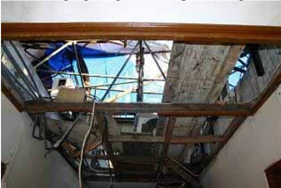
Damage to roof system above top story (some column rebar were not anchored to beams)
