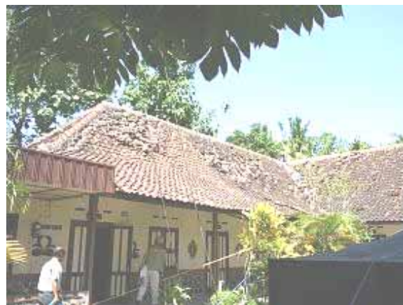
SD Tempel at Bambanglipuro / Heavy damage to URM wall and fallen ceiling boards
