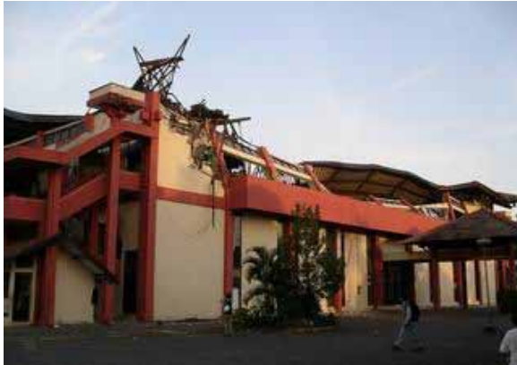
Amongrogo Sport Center / Collapsed roof system associated with column failure underneath
