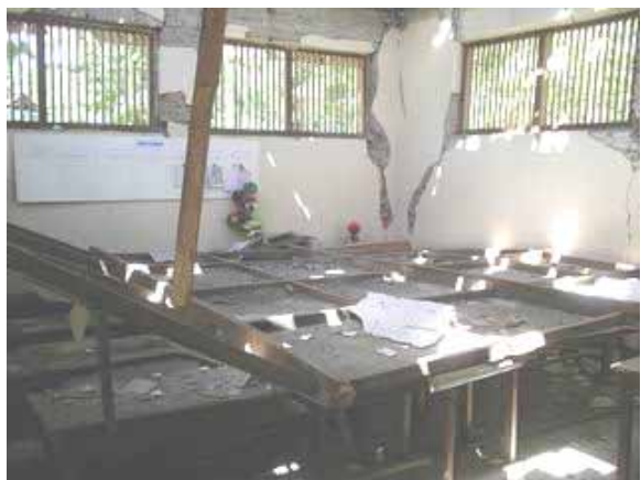
SD Tempel at Bambanglipuro / Heavy damage to URM wall and fallen ceiling boards
