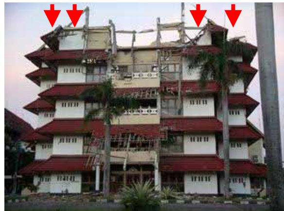
5 story building with 4 URM wall frames
