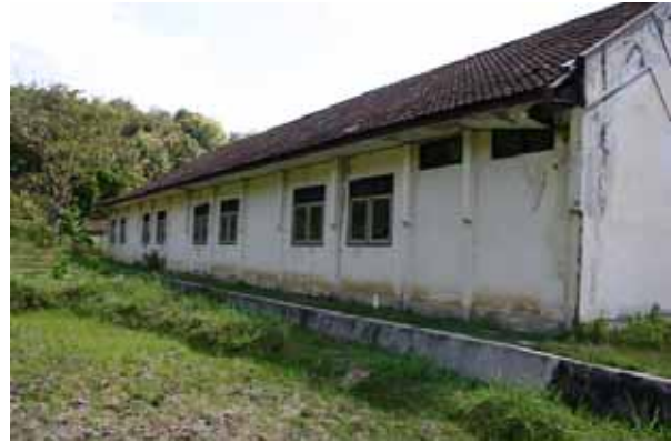
South side of building #1
