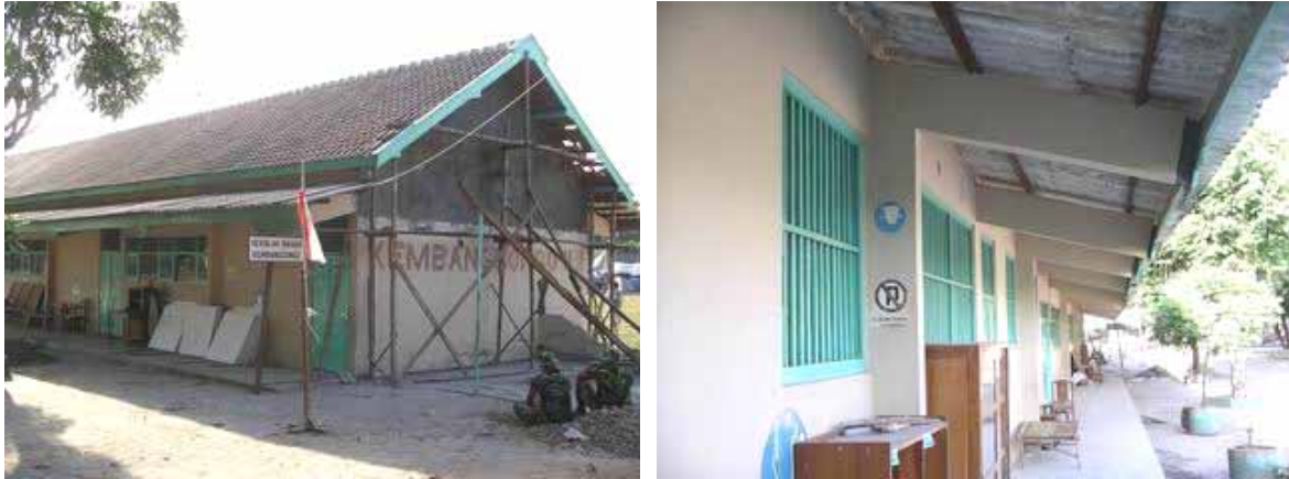
SD 2 at Kembangsongo / No major structural damage found in the building
