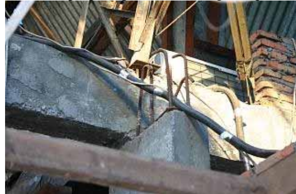
Damage to roof system above top story (some column rebar were not anchored to beams)
