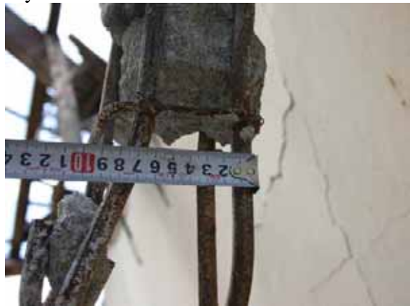
SD Pesu / Exposed rebars in a column supporting roof system above
