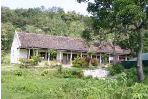
Building #1 : URM with RC columns
