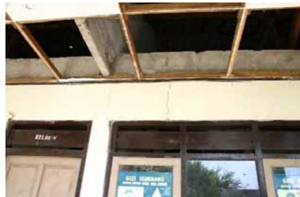
Building #1 : RC column and beam
