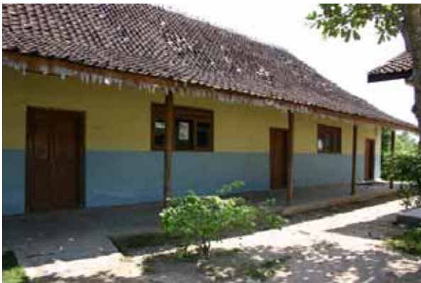
Building #2: Stone masonry structure
