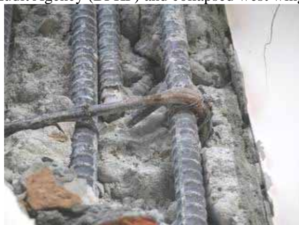
135-degree hooks in a column
