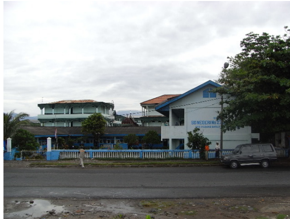
Fig. 9. Multistory school buildings with balcony directly accessible from the ground level can be primary candidates for practical tsunami shelters.
