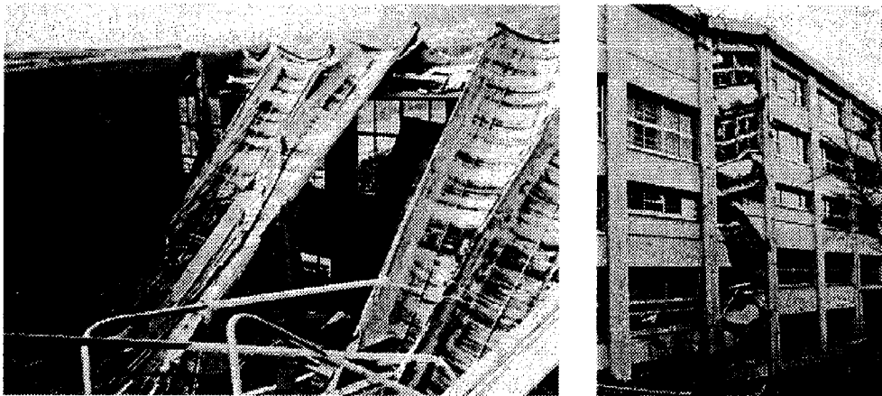
Figure 1. Seriously Damaged Schools due to the 1995 Kobe Earthquake
