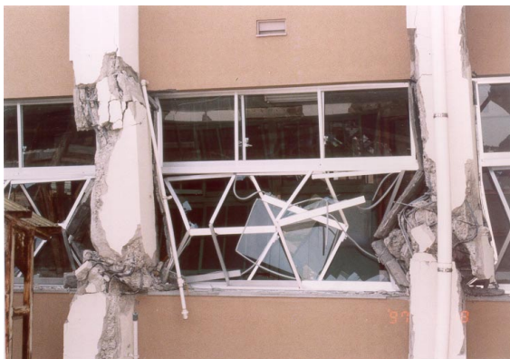
Damage class V
