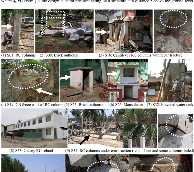
(10) T09: RC fence columns of Navy Base (rebar fractured)
